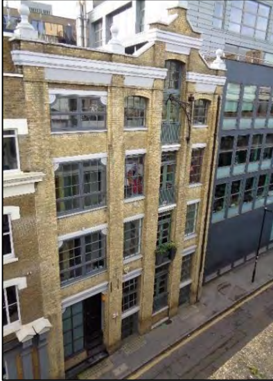
Figure 30: 17-18 Clere Street (western elevation)
