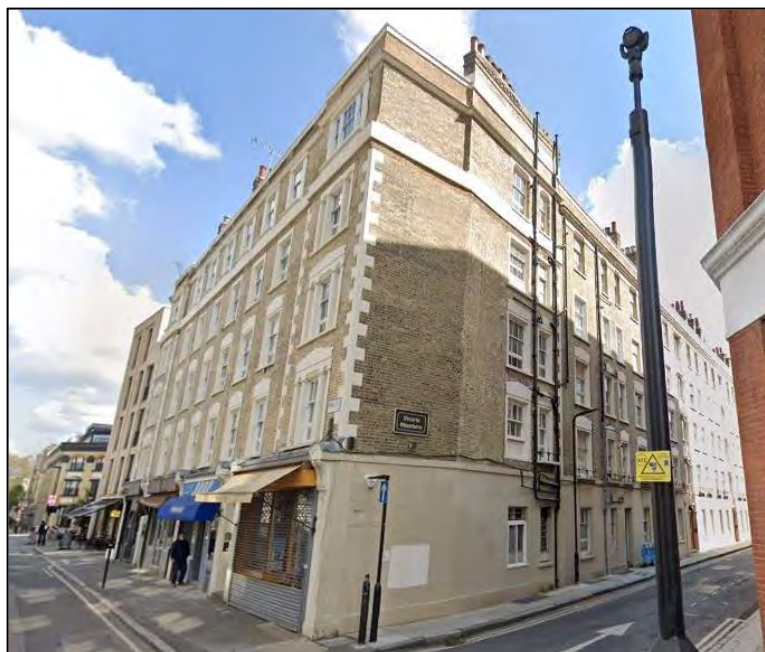
Figure 33: The front and side elevations of 54 Paul Street
