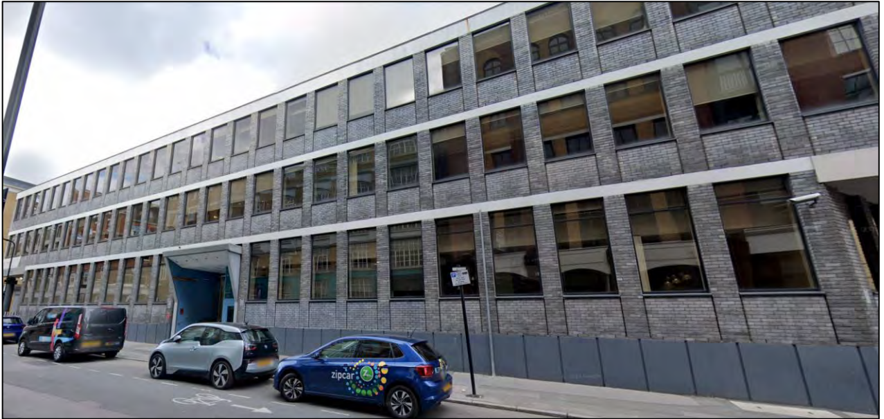
Figure 6: Paul Street elevation, looking south
