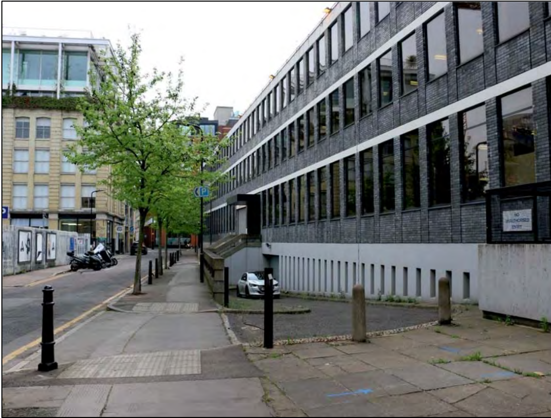
Figure 8: Clere Street elevation, including vehicular ramp to lower ground, looking east
