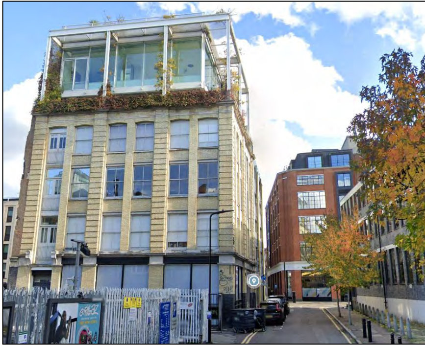
Figure 31: 17-18 Clere Street (western elevation)
