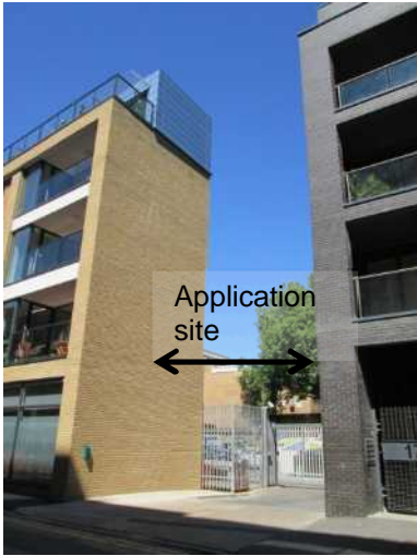
Existing entrance from Pear Tree Street
